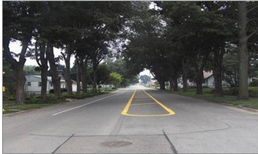
Figure 6.9 Wide centerline median striping.
