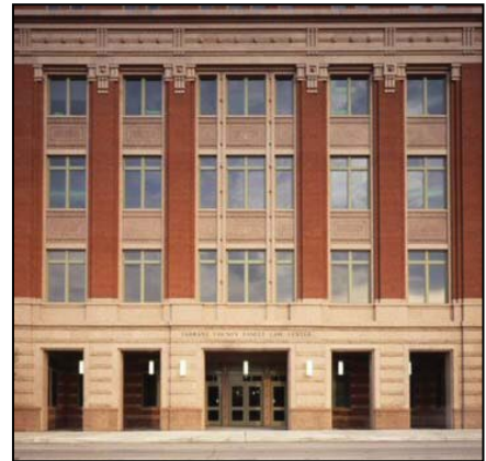
Figure 5.35 No single material covering more than 80% of front façade
