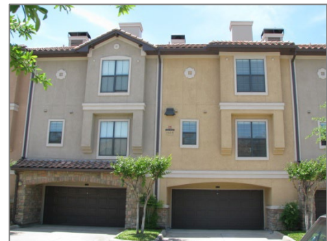
Figure 5.23 Garages integrated into building.
