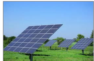
Figure 3.1 Ground-mounted solar energy system.
