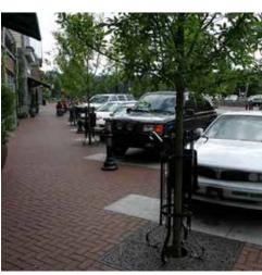
Parking constructed with pervious material
