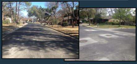
New asphalt pavement is laid for the entire width of roadway. Concrete pads are placed around manhole lids. Roadway striping is restored if necessary.
