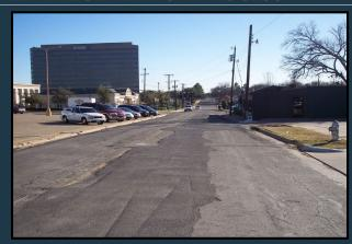
The street is repaired with temporary asphalt patches after installation of utilities. Curb, gutter, and driveways are replaced.
