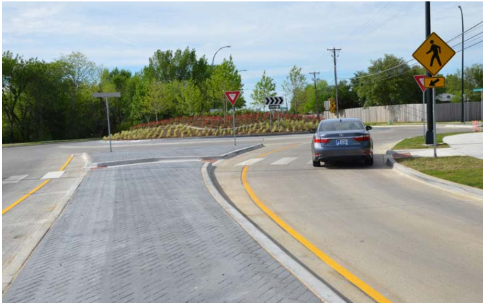
Tri-schools Project Roundabout
