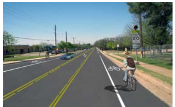
Bike lanes, like those shown in this rendering, include striping that designates part of the road space for cyclists
